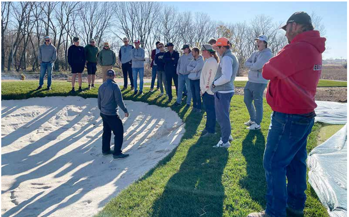
Eric Leonard at TPC Wisconsin talks about bunker construction to the students in the Turfgrass Apprenticeship Program.
