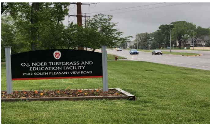
The road construction is complete! The new sign and entrance to the O.J. Noer Facility.
