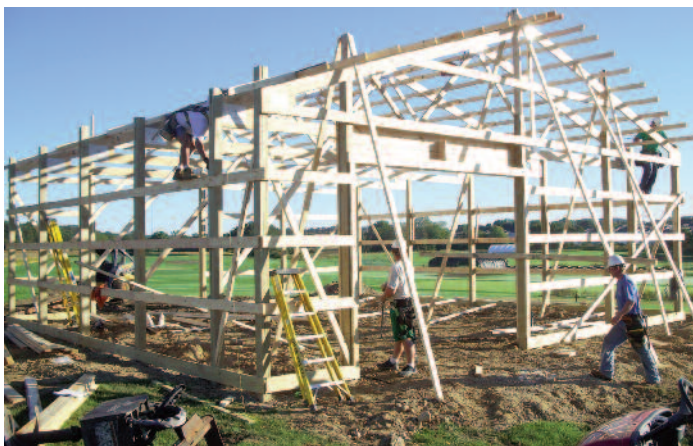
All this work was completed in one day
