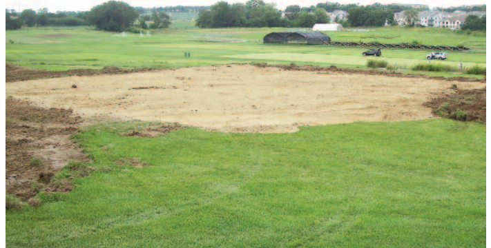
36 x 36 foot building pad site
