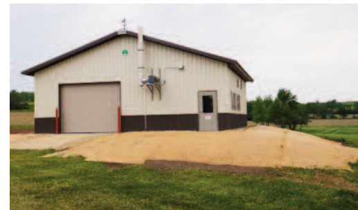
Surrounding slopes contoured, seeded, then protected from erosion with Futerra blankets
