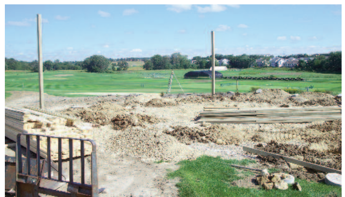
Start of building assembly
