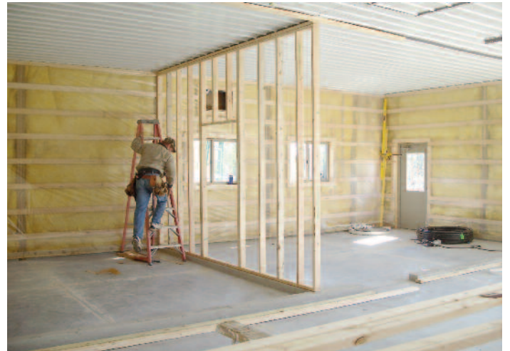
Fred Turner building interior walls
