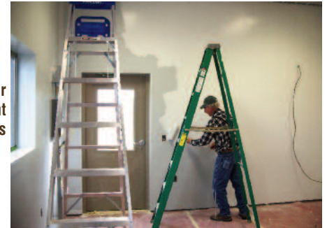
Noer employee Walter Thieszen helping paint interior walls
