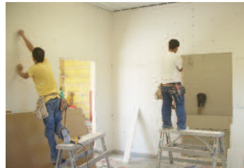
Dry wall finishing
