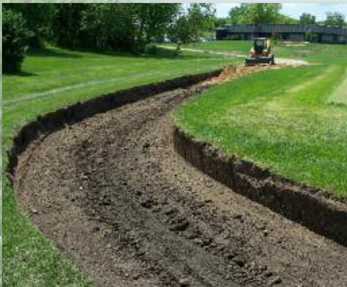
Building of service road to access new bridge
