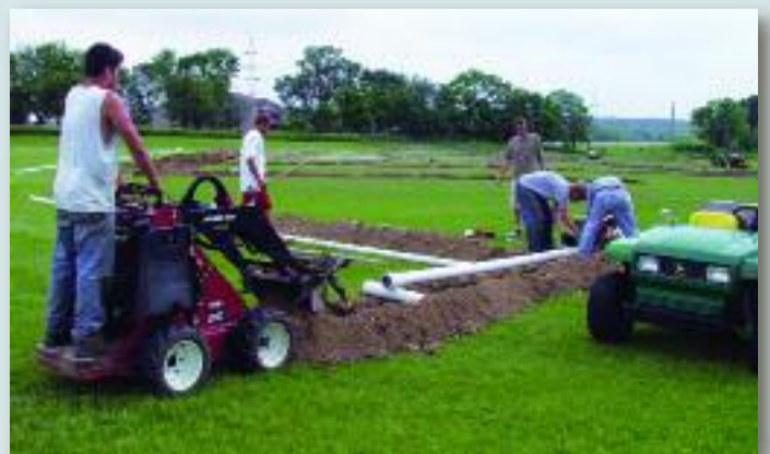
Installing irrigation to NE quadrant
