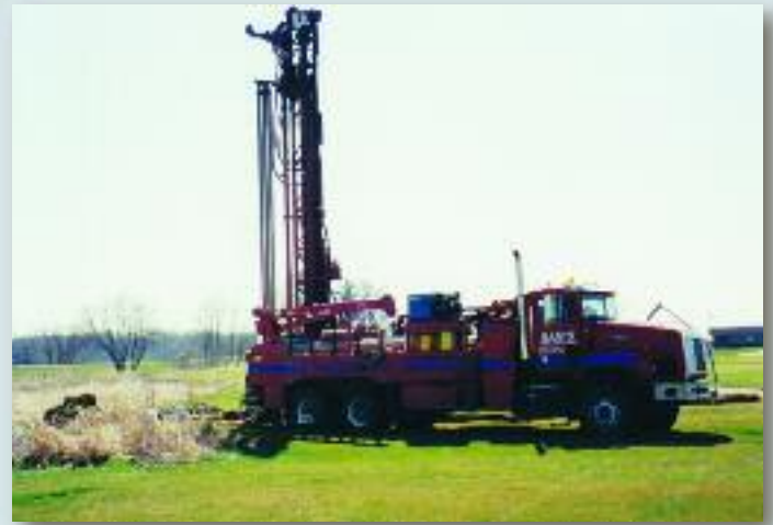
Digging new high capacity well
