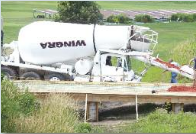
Pouring concrete bridge
