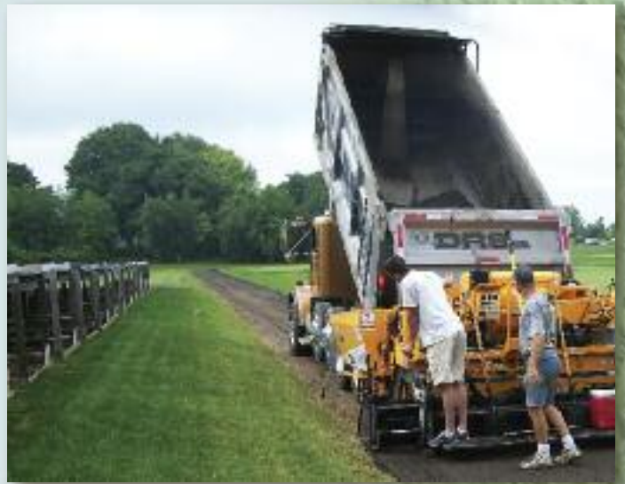
Recycled blacktop paving of service roads
