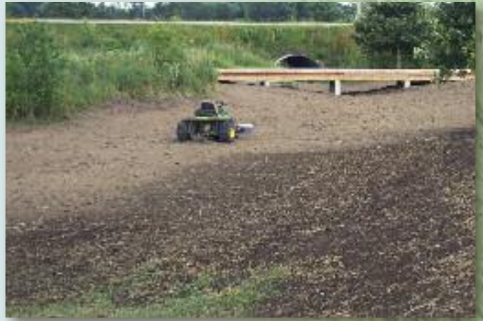
Seeding drainageway around bridge
