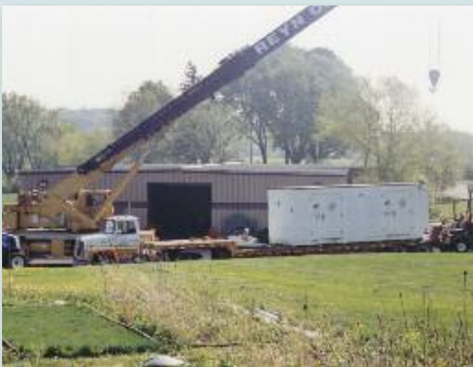
Delivering temporary pesticide storage trailer
