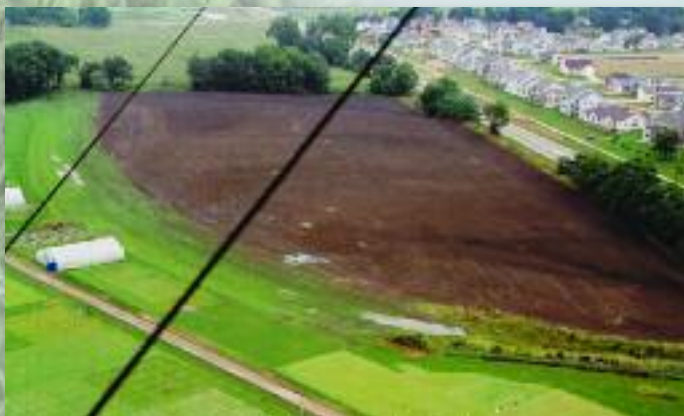
NE quadrant including enlarged drainageway after reshaping and before seeding
