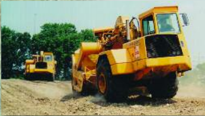
Bruce Company's scrapers and dozers shaping 10 acres NE quadrant addition
