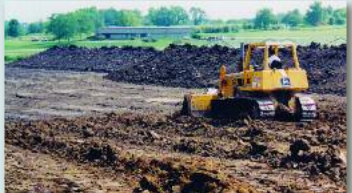
Bruce Company's scrapers and dozers shaping 10 acres NE quadrant addition
