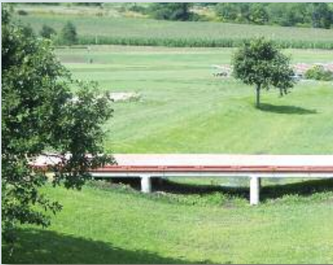
New drainageway and bridge
