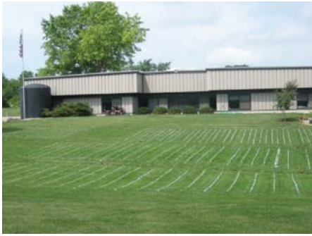
(3) Complete plot area with drip irrigation laterals marked prior to installation. Noticeable are different drip lateral spacing.
