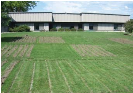
(4) Plot area during drip lateral installation.
