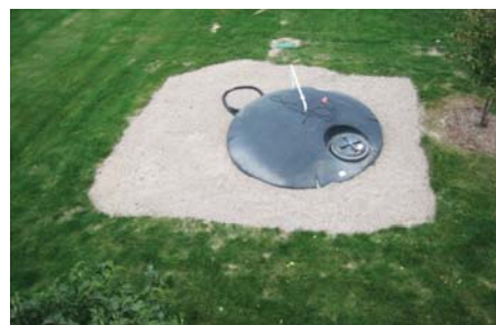
(2) Below ground tank located near the Northeast corner of the building. Visible are the access hole and water outlet. Subsurface collection conduit is not visible.
