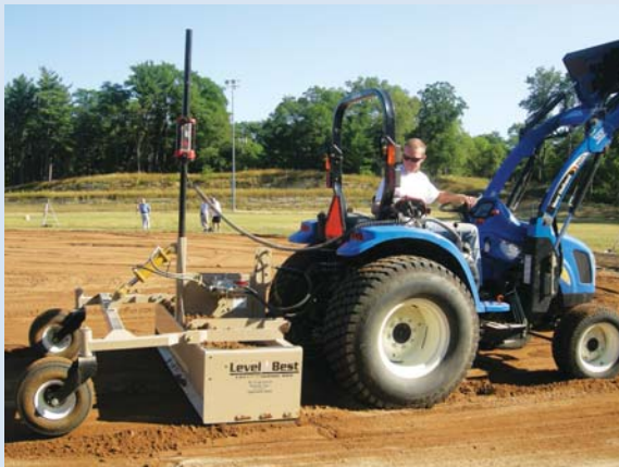
Josh Viet from Midwest Athletic Fields uses his laser grader to level the new infield.
