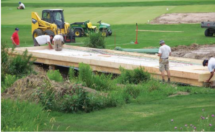
Building the forms for the concrete deck
