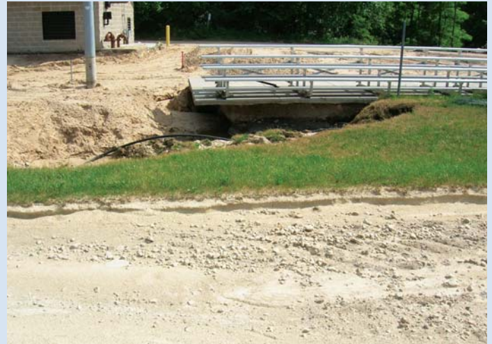
The damage to the third baseline and bleachers from the rushing waters.
