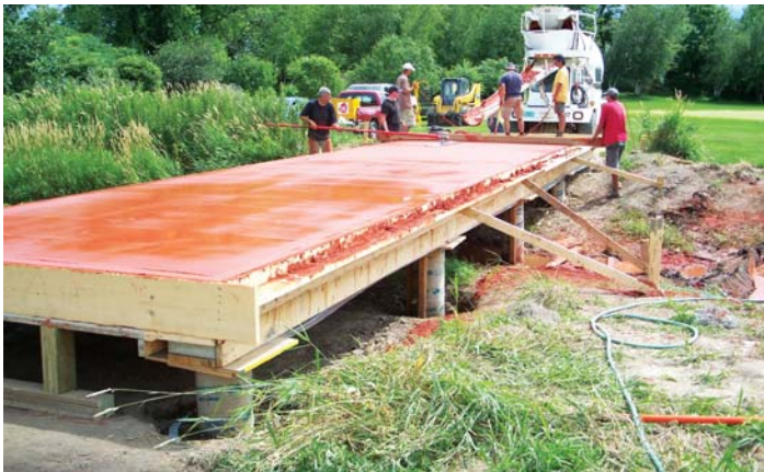
Pouring the concrete deck
