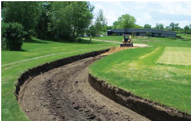
Constructing the access road to the bridge
