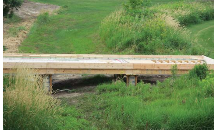
The deck is almost ready for concrete
