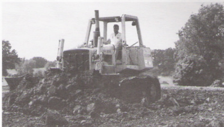
Bob Theodozerguy starts to reinstall the topsoil.
