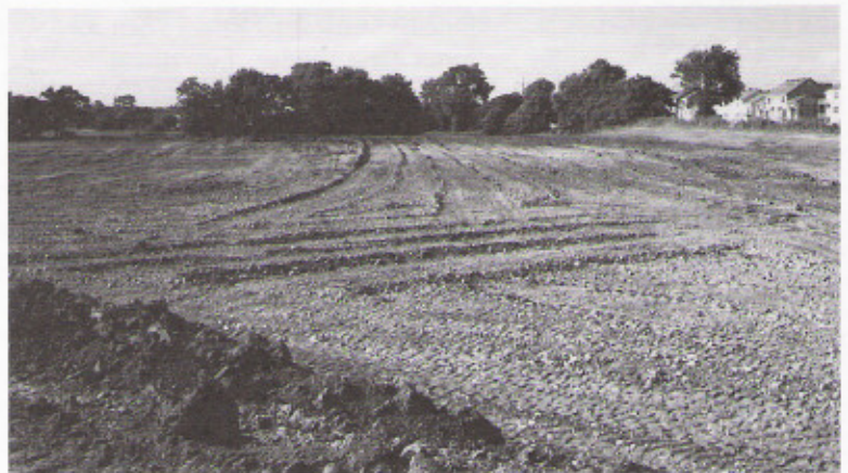
Subsoil is contoured to specifications and ready for topsoil.
