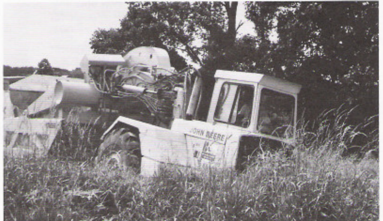
Scrapers heading into the work zone.
