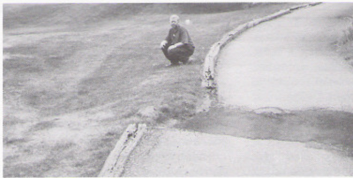
This land shift made the cart path and surrounding area slump.
