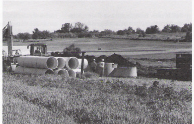
Sewer pipe to serve new subdivision of Madison.
