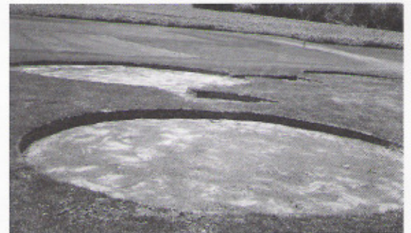
First step was to excavate 6 inches of soil...
