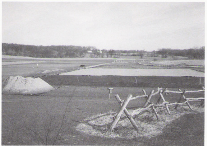
10,000 square feet of USGA and 5,000 of native soil green are nearly completed and ready to seed.
