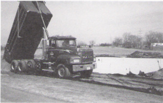
Greensmix trucks delivering the rootzone mix.
