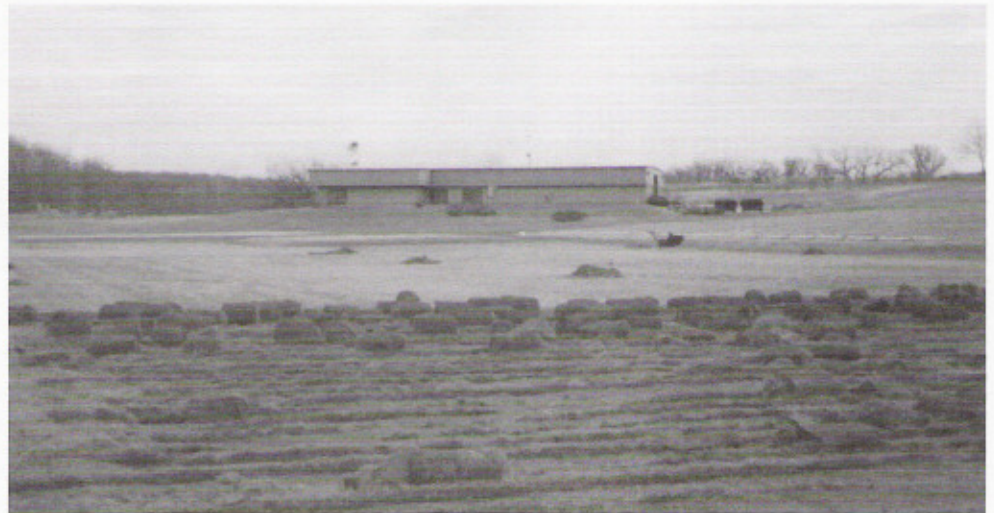
Phase one — stripping the sod away.
