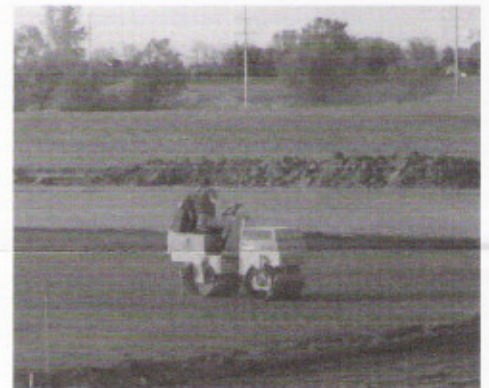
Finishing touches before seeding.
