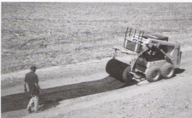
Laying out the big rolls for a roadside job.
