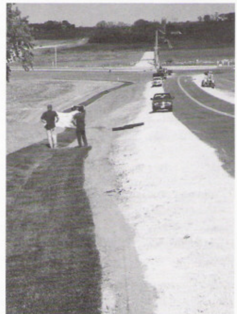
Instant roadside erosion control.
